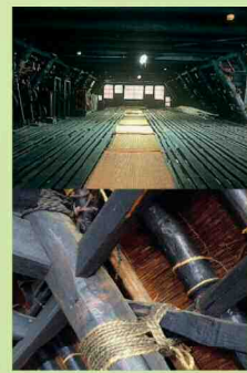
Gassho-zukuri are constructed using only rope and timber; no nails or metal fittings are used.
