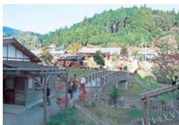
Kunma Suisha Village Rest Station
